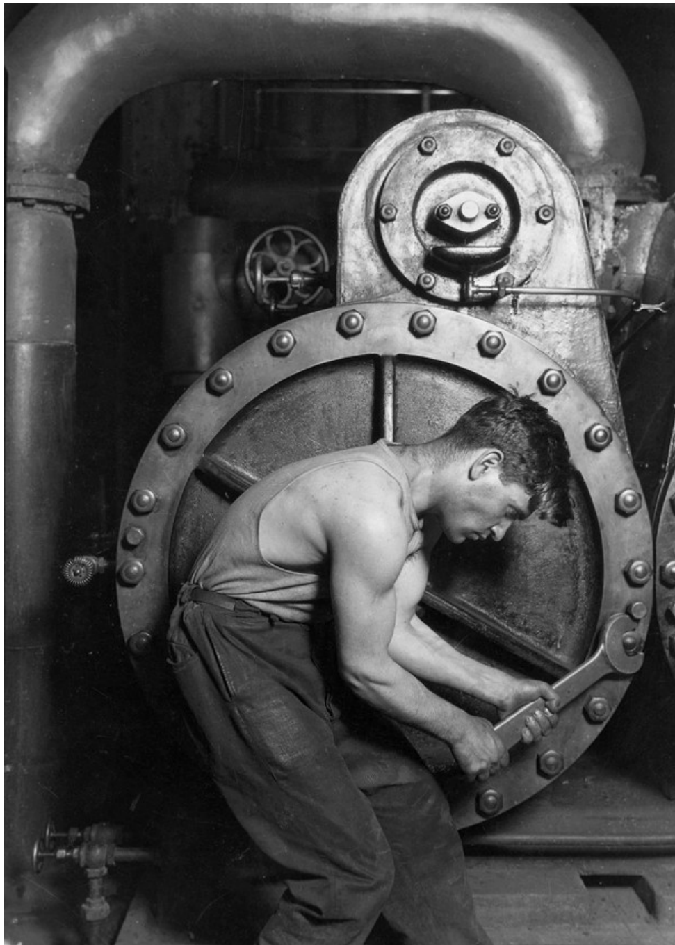
Lewis Hine, Powerhouse Mechanic or The Steamfitter, c. 1920
